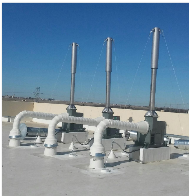
Typical Class II BSC Exhaust System
